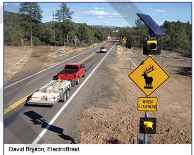
Figure 45. Animal-activated warning light in Payson, AZ, triggered when large wildlife are detected near the road. Source: U.S. Department of Transportation, Federal Highway Administration article, Advances in Wildlife Crossing Technology , by Mary Gray.
